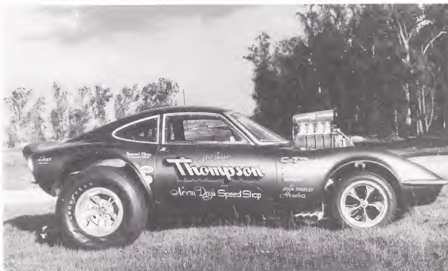
Junior Thompson's Opel GT. It was quite a trick to shoehorn a supercharged Chrysler into the engine compartment of such a tiny car. (Courtesy Museum of Drag Racing)
