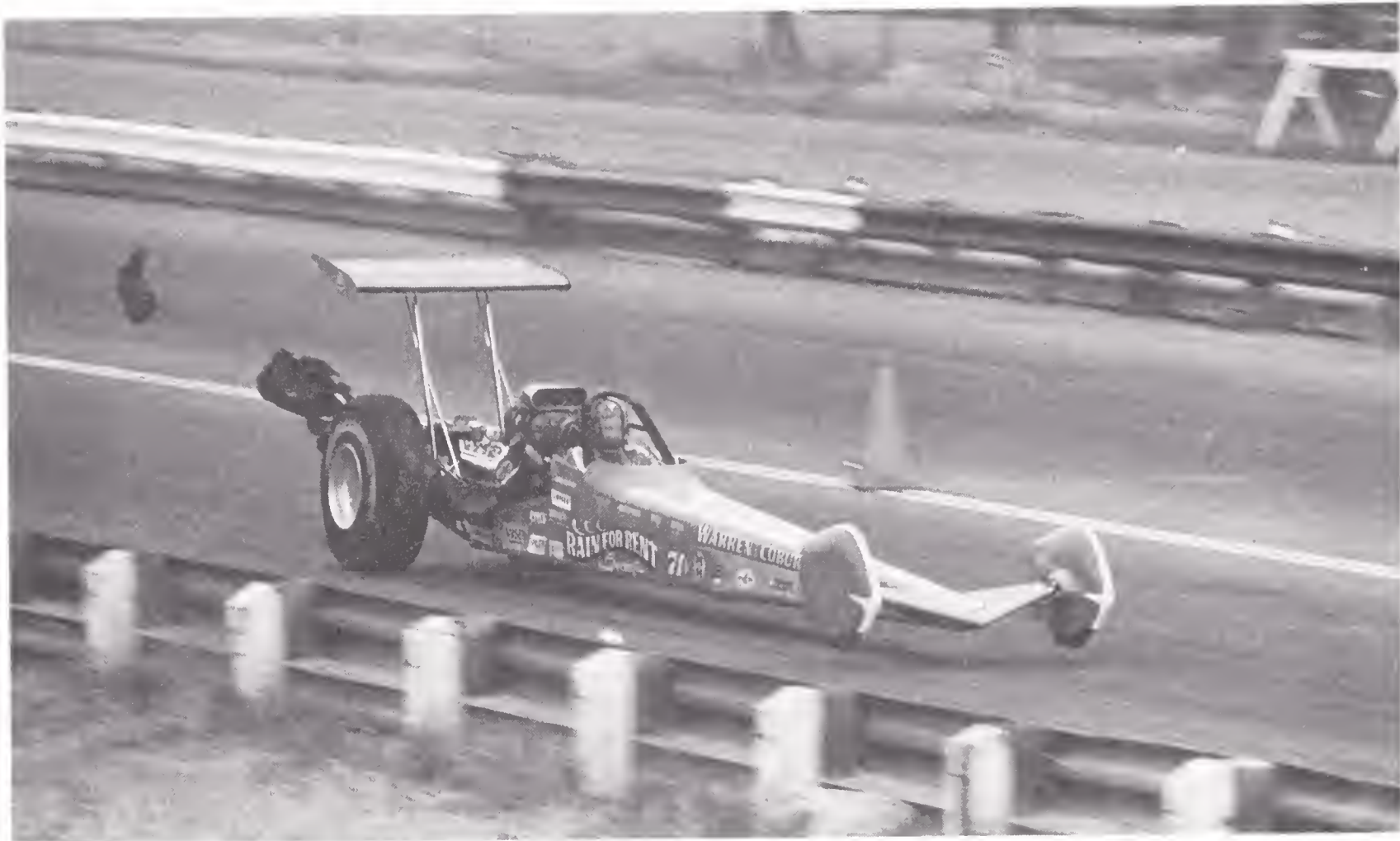
A mid-engine fueler outfitted with pants on the front wheels; most racers flirted with these devices only briefly, and NHRA later prohibited them. In this photograph driver James Warren has just hit the parachute release while still under power with his wheels in the air, and the spring-loaded pilot chute is pulling the main chute out. (Photograph by John Shanks)
