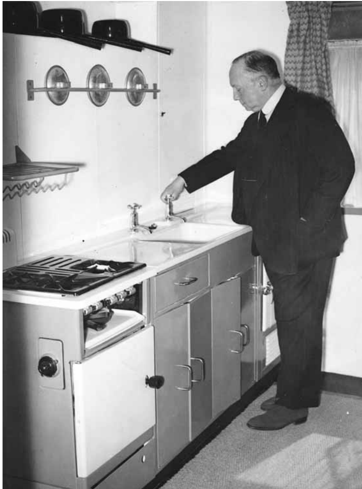
The British Minister of Health, Lord Portal, in 1945 posing for a publicity photograph in the standard kitchen that the British government built for the 154,000 temporary prefabricated bungalows constructed after World War II. Lord Portal's name became synonymous with the prefab, which owed a great deal of its popularity to the ingenious design of this kitchen. Source: Architects' Journal (1945).
