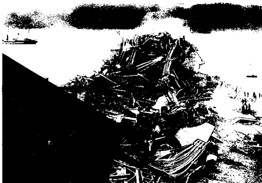
Figure 28. The building (a) of the Quebec Bridge spanning the St. Lawrence River. Its collapse (b) on August 29, 1907, came to symbolize faulty design of male character and professional ideals in several plots engineered by women novelists. Photographs both courtesy of Division of Engineering and Industry, National Museum of American History, Smithsonian Institution, Washington, DC. (neg. 91-6990 and 91-6981).
