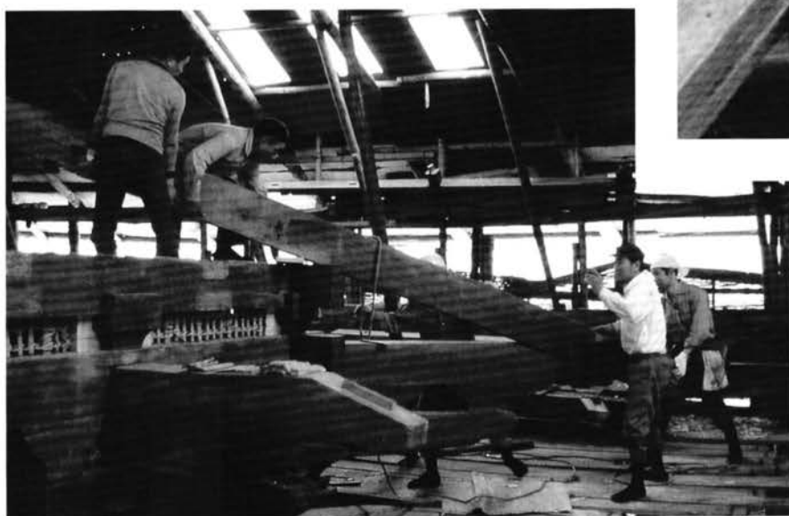
Figs. 5.36–5.39 Hakkiji pagoda during restoration
