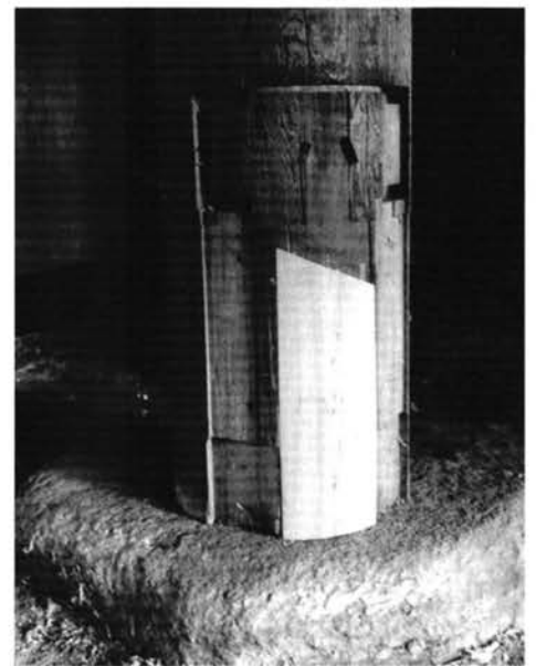
Fig. 5.32 Hokkiji pagoda, cavities in a column on the ground floor
