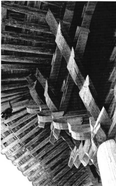
Fig. 5.50 Timber pagoda at Yingxian, bracketing cluster, third story
