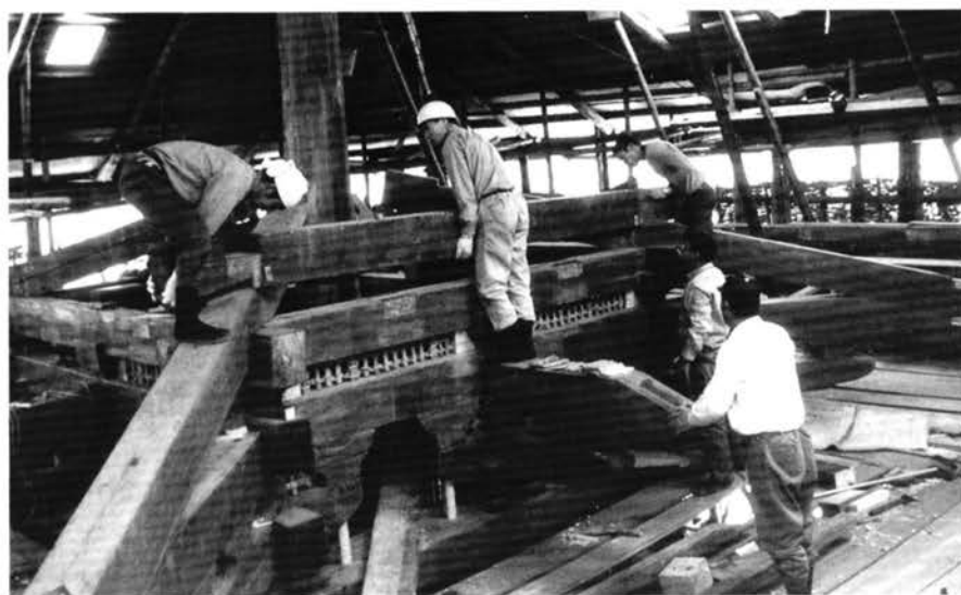
Fig. 5.39 Workers lowering longitudinal beam onto ang beam
