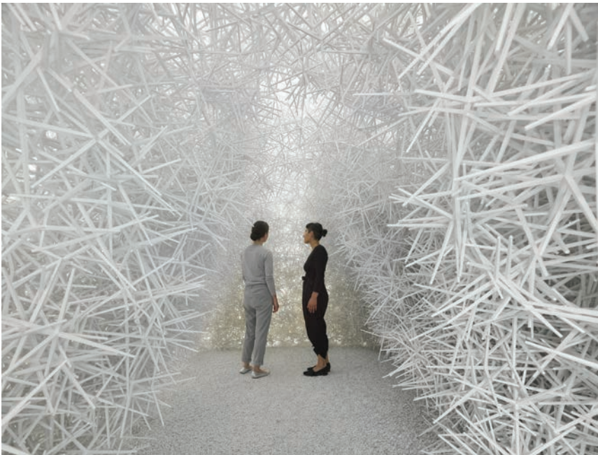
11.5 ICD Aggregate Pavilion 2018. Karola Dierichs, ICD, University of Stuttgart. For the ICD Aggregate Pavilion 2018 convex and non-convex particles were combined. The convex particles served as a formwork for the interlocking, non-convex ones. The particles' dimensions are in the range of circa 10 to 30 centimeters. After the entire structure had been poured in situ, the convex particles were removed from the inside of the pavilion and a stable vault formation remained standing. Courtesy of Roland Halbe
