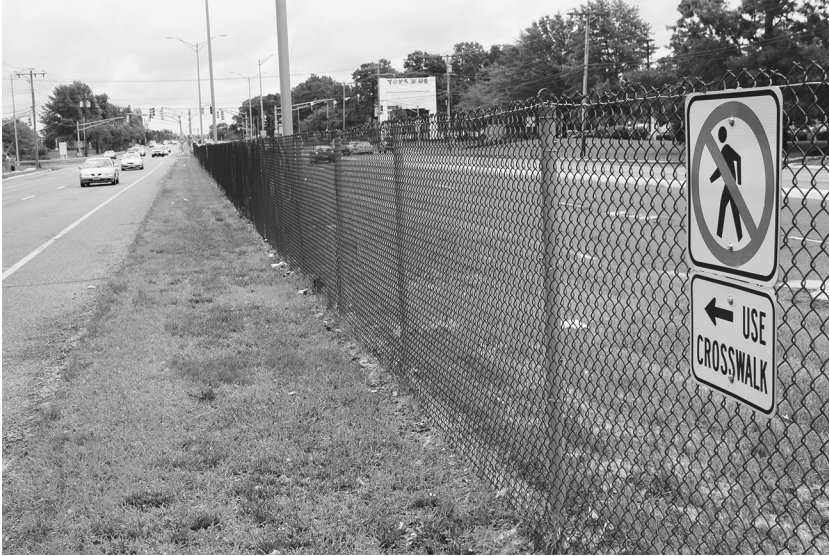
FIGURE 3.6. A symbolic and material fix. In this location on Black Horse Pike, a bus stop is situated on the westbound side, across the highway from a large shopping center. An intersection with a crosswalk is perhaps a hundred yards away. The sign reinforces the message that is conveyed (and physically enforced) by the fence. Together, these objects encourage pedestrians to trade convenience for safety, while preserving the priority that drivers hold in the programming of this place.
