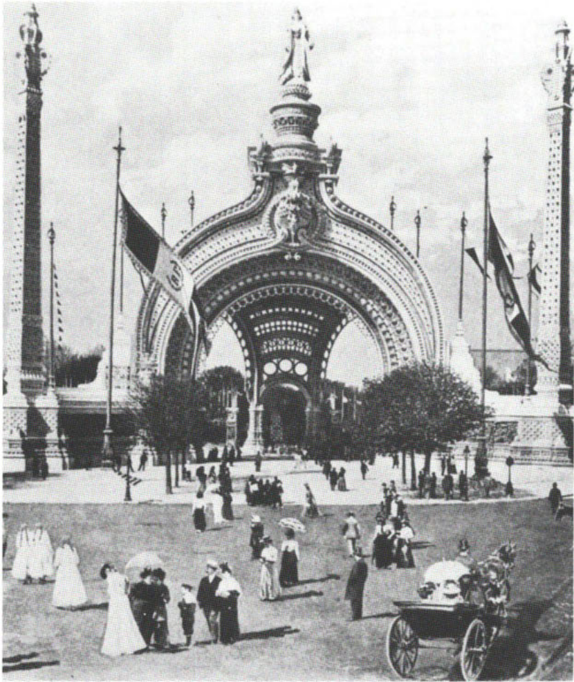
10. The Monumental Gateway (La Porte Binet) on the Place de la Concorde during the 1900 exposition, Paris. The Gateway consisted of one high entrance arch and two smaller arches, under which were located fifty-six ticket offices. Above the triangle formed by the three arches was a dome, and on top of the dome stood the statue of La Parisienne. The slender pyramid-shaped minarets on either side of the arch were studded with crystal cabochons and were lit at night from inside. The overwrought polychrome decorations of the Gateway seemed the creation of a mad jeweler. (Illustration from Paris 1900 by Franco Borzi and Ezio Godoli, published by Rizzoli International Publications, New York.)
