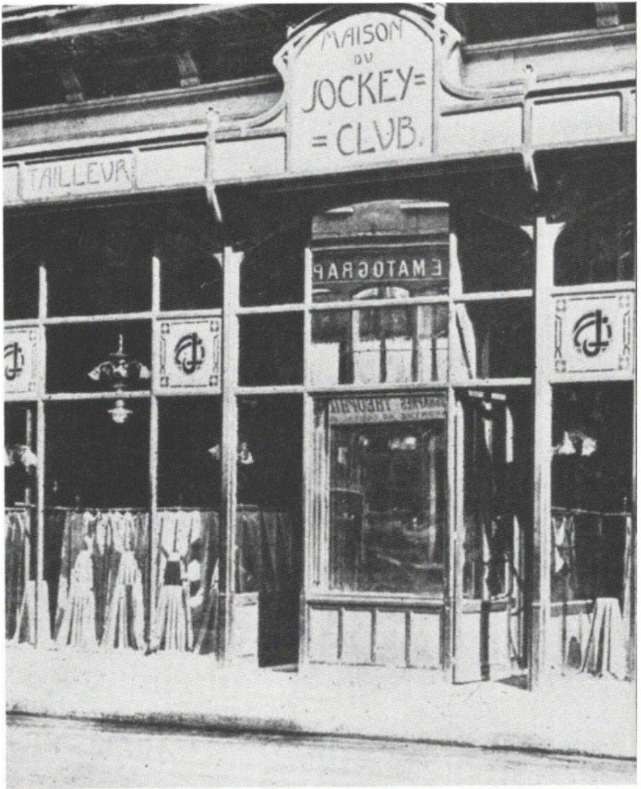
11. The Maison du Jockey Club, a tailor shop on the Boulevard des Italiens. The Jockey Club had long been a fashionable haunt of Parisian dandies, and this shop assumed the name in order to lend prestige to the business. The façade, an example of the application of Art Nouveau motifs to commercial establishments, demonstrates the creative use of electrical lighting by stores: the names and signs are written on glass lit from behind. (From Architectural Record , vol. 26, no. 2, August, 1909: 116. Courtesy of Architectural Record .)
