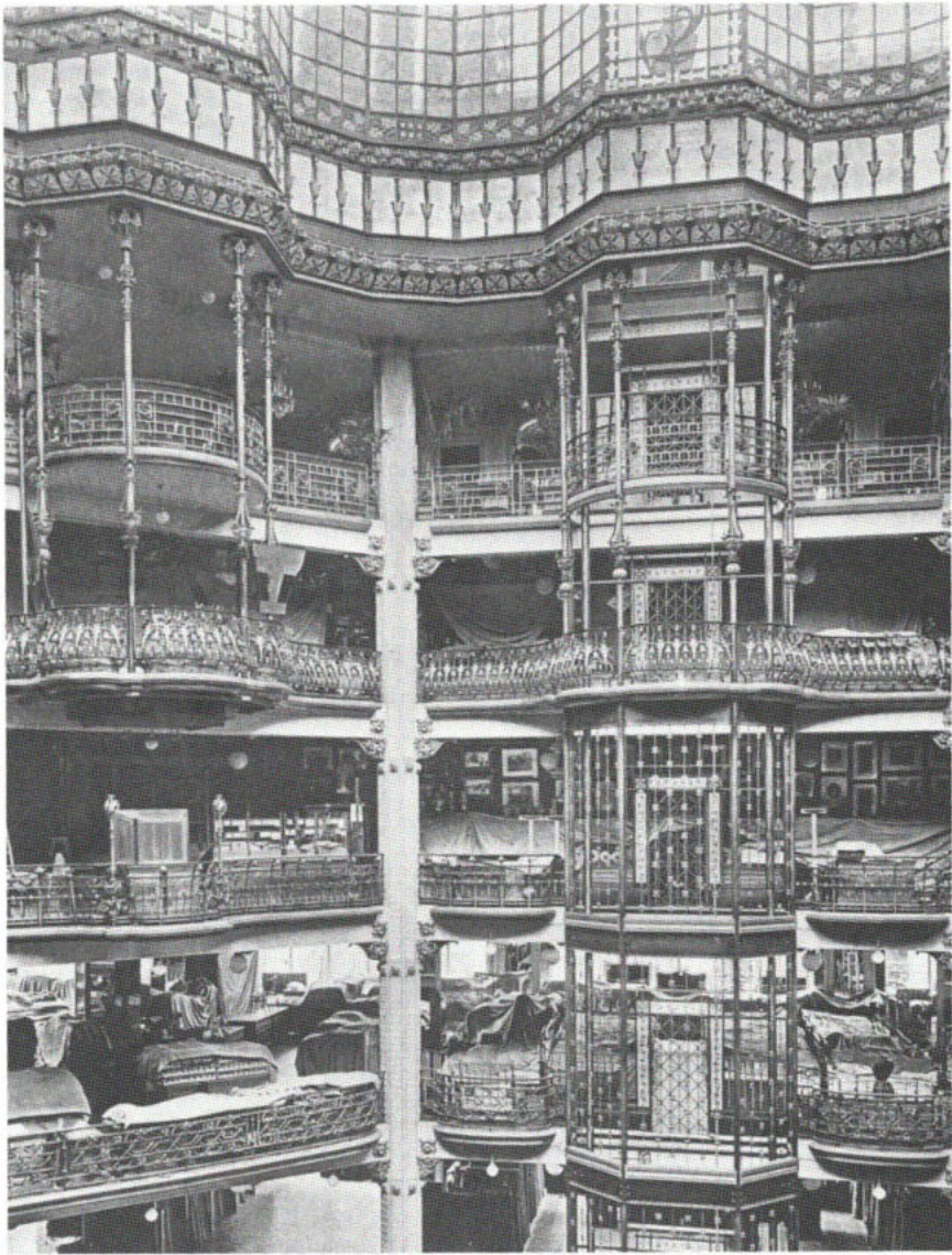
18. The Grand Hall of Binet's addition to Grands Magasins du Printemps, as it appeared in 1911. Instead of hiding the elevators in an inconspicuous place, as previous department-store architects had usually done, Binet made three large elevators prominent decorations of the Grand Hall, which was seven stories high. An admirer of Binet's design explained, "The intensity of life no longer permits the shopper to pass slowly from one level to another by a staircase; the shopper wants to be carried instantaneously from the ground floor to the highest story, without fatigue, with a speed equal to that of his automobile." (Photograph from L'Architecte , 1911, pl. 10.)
