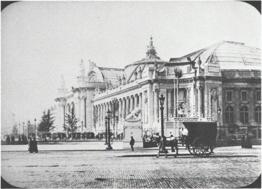
5. Exterior view of the Grand Palais, built for the 1900 exposition and later used for a wide variety of public events, including the Salons de l'Automobile. The facade of stone, featuring an Ionic colonnade before a mosaic frieze, is architecturally conventional. Far more striking (especially when the Grand Palais is viewed from a distance) and more innovative are the steel and glass domes forming the roof of the main part of the building. (Lantern slide in the Rotch Visual Collection, M.I.T.)
