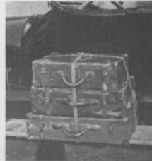
Having four straps ending in clasps which screw to the upper surface of the running board and brought to a top leather disc, this guard holds from one to three full-sized cases. Price, $3.50
