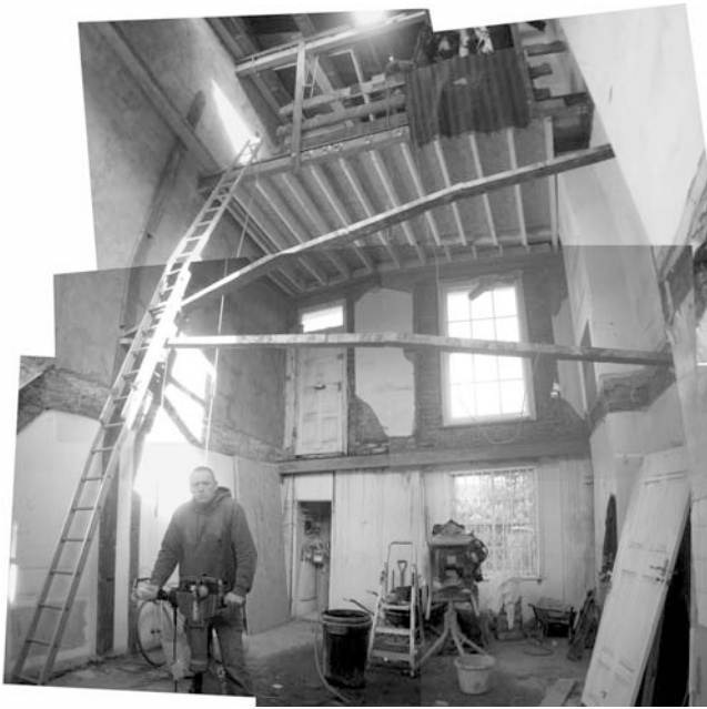
Figure 5.2 'Site Progress', Victorian conversion, Hackney, 2009
