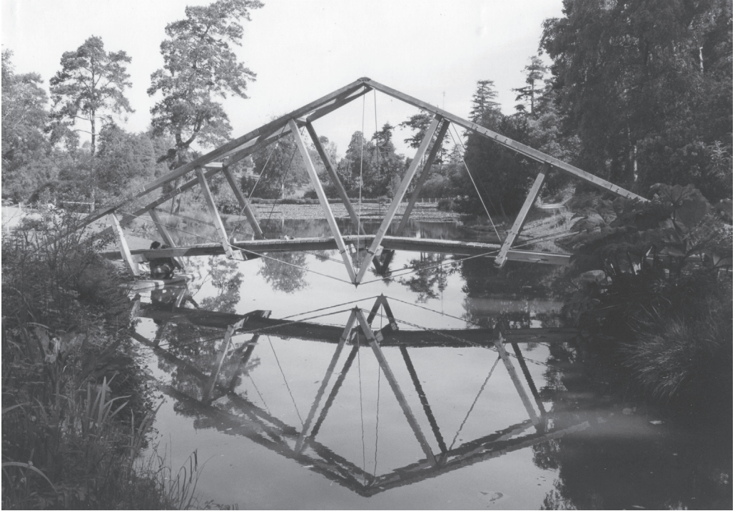
Figure 4.3 Richard LaTrobe-Bateman, Diamond Truss Bridge , 1995. English oak and galvanized steel. Engineered by Mark Lovell. National Pinetum, Bedgebury, Kent. Courtesy of the artist.
