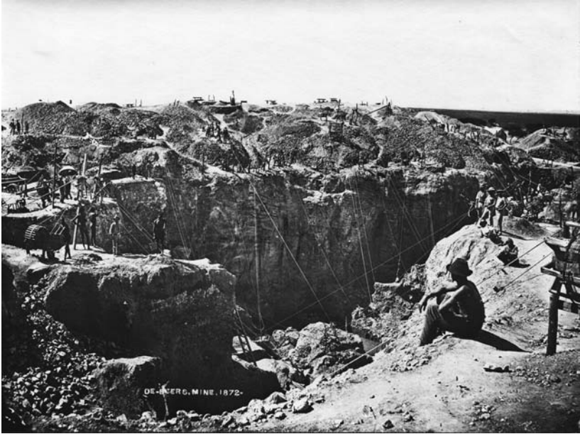
2.1. DeBeers Mine, Kimberley, ca. 1872. This figure illustrates the early working of one of the two biggest open-pit diamond mines, the other one being the Kimberley Central Mine on the other side of town. Note that various small claims have gone to different levels of the mine. Miners are using a system of winches and ropes to haul out the earth before sorting it nearby. Photo courtesy of the McGregor Museum, Kimberley. MMKP 4447.
