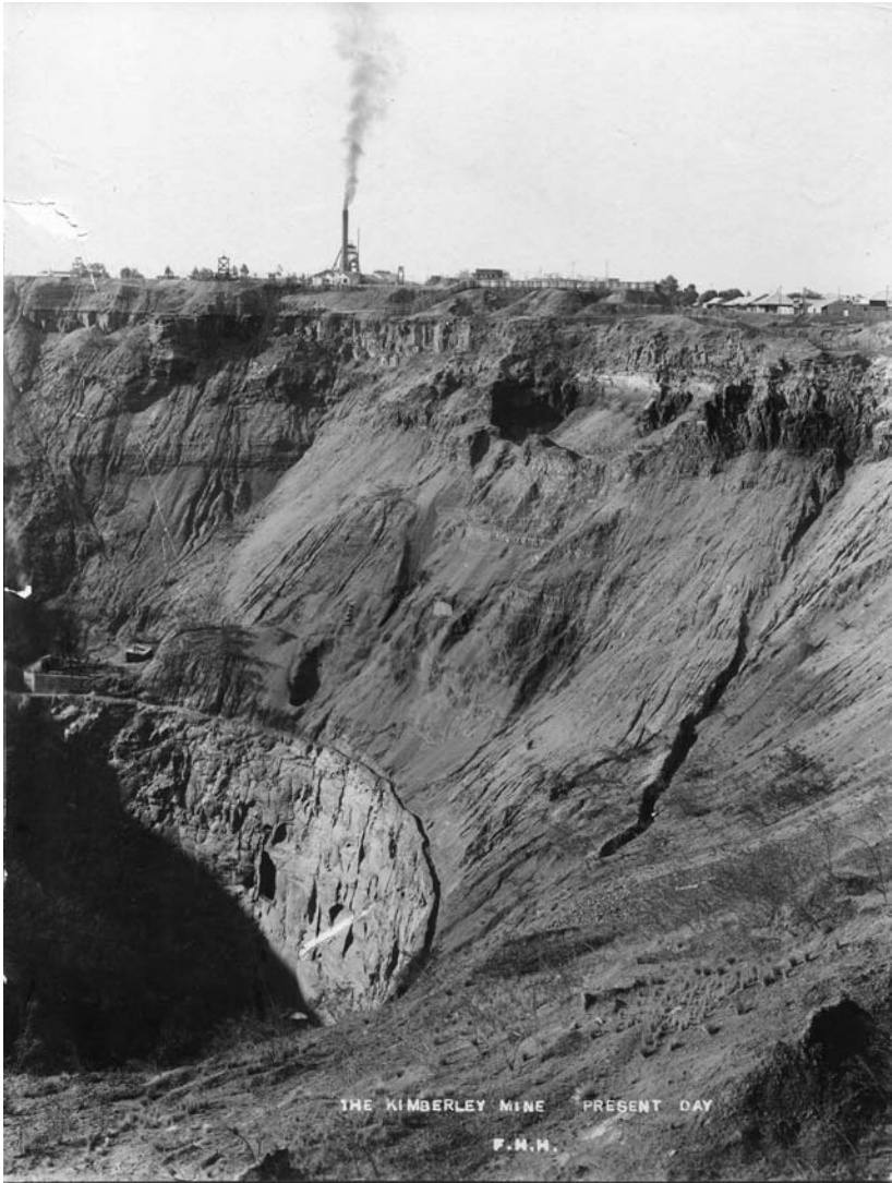
2.2. Kimberley Central Mine, ca. 1895. The open pit, known as the “Big Hole,” was excavated by 1888. Note the strata of earth as well as the cylindrical shape of the Kimberlite pipe. At this point in time, diamond mining is taking place in tunnels that lay beneath the open pit. Photo courtesy of the McGregor Museum, Kimberley. MMKP 5334.
