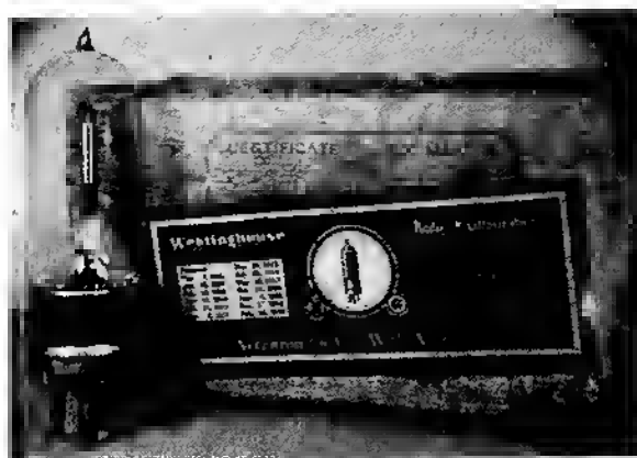
Fig. 16-5. Westinghouse E. & M. Co.'s Aeriotron WD11, with packing carton. Note the lime getter on the press.
