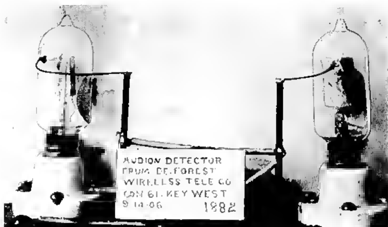
Fig. 4-11. Panel mounting two-electrode Audions installed at Key West, 1906.
