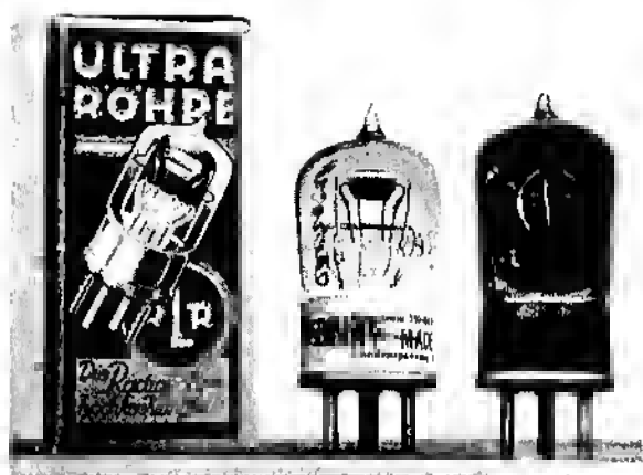
Fig. 21-42. Ultra UL550 (left) and U60 (right) tubes, with carton.
