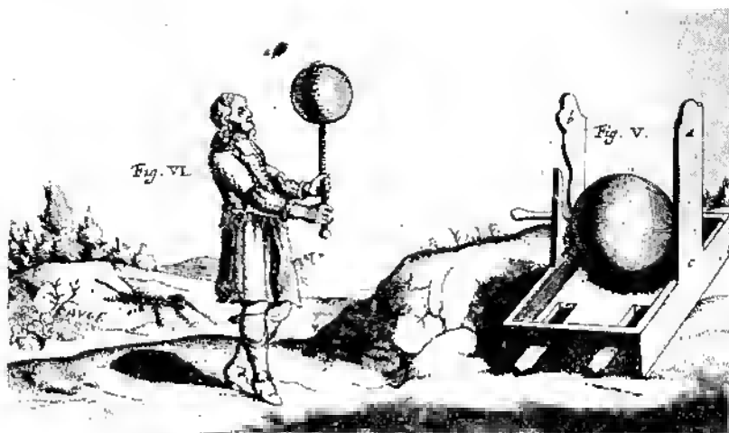
Fig. 1-1. Right: Otto von Guericke's "electrical machine." Left: operator using charged sulfur ball to repel feather. (Reproduced from Experimenta Nova Magdeburgica de vacuo spatio , Amsterdam, 1672.)
